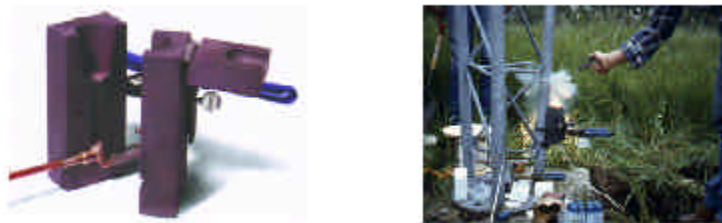
FIGURE 23-48 EXOTHERMIC WELDING MOLD (LEFT) AND PROCESS (RIGHT)
