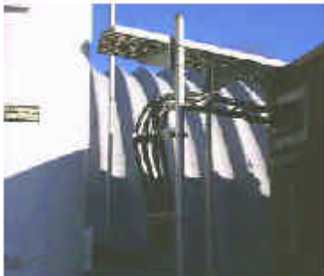
FIGURE 23-20 Example of Ice Bridge Isolated from the Tower
