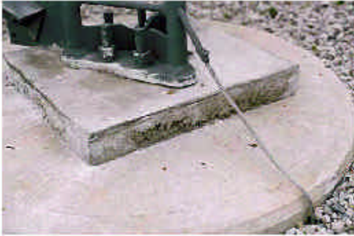
Figure 23-21 Self-Supporting Tower Leg Grounding
