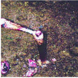
FIGURE 23-49 COMPLETED EXOTHERMIC WELDS IN TRENCH AND ON TOWER
