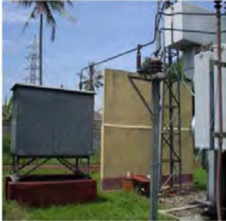
Gambar 5.6 Resistor Jenis Logam
