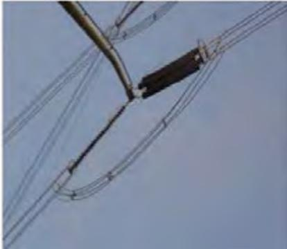
Gambar 4.33 . Tension clamp 5. Suspension clamp
