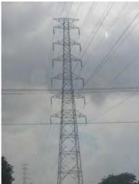
Gambar 4.8 Tower 4 sirkit tipe suspensi tipe tension
