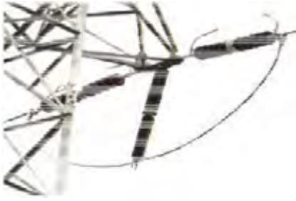
Gambar 4.32 Tension clamp
