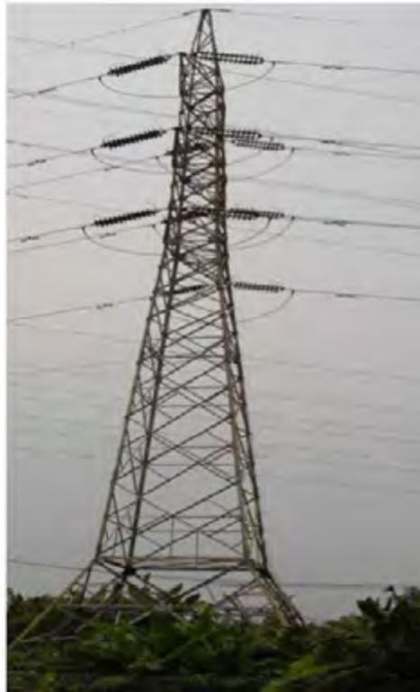
Gambar 4.11 Tower 2 sirkit tipe tension
