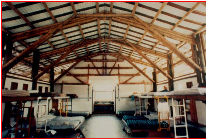
Gambar XI-40, Rangka Atap Bambu
